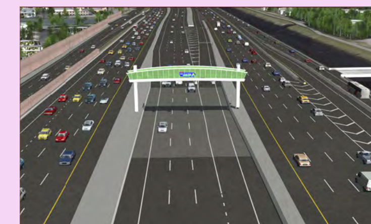
Open Road Tolling Express Lanes Gantry
