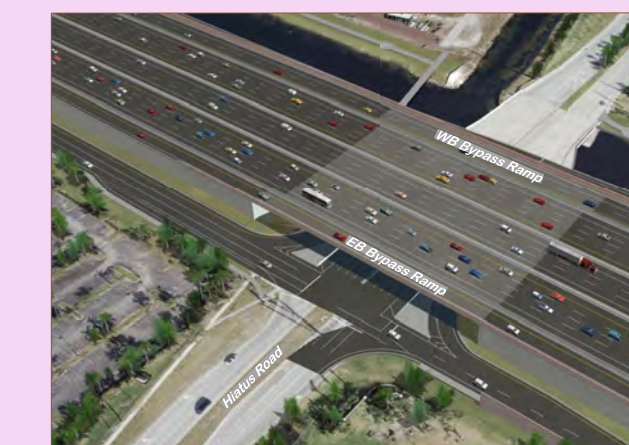
Bypass Ramps at Hiatus Road
